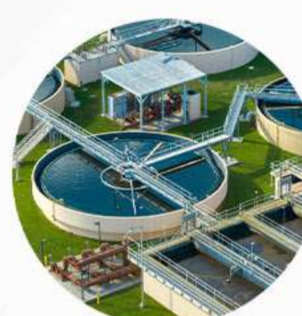
Water & Industrial Water Treatment
