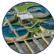
Water & Industrial Water Treatment
